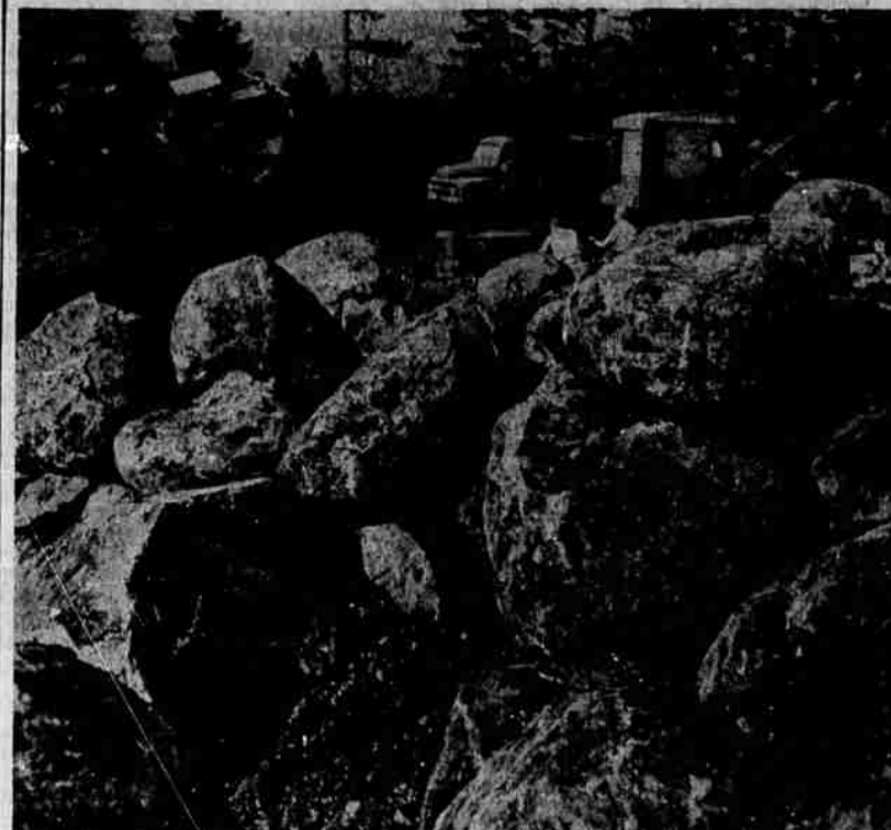
Boulders in large numbers, some of them as much as 10 feet in diameter, were encountered by workmen engaged in lowering the grade for the new elementary school on South 12th Street.
