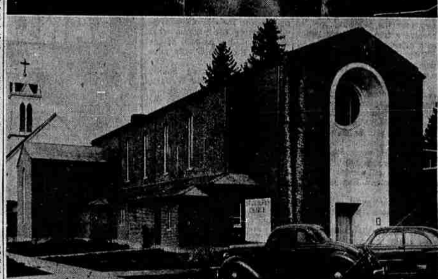
Top: View of interior from sanctuary looking through the nave of New St. Joseph's Catholic church. Oak pews carry a platinum finish. Seating capacity on the main floor is 700. 50 more can be accommodated in the balcony. Lower: Exterior view of new church to be dedicated on Thursday morning, St. Joseph's day, with cornerstone ceremony and pontifical mass read by Most Rev. Edward D. Howard, archbishop of Portland.
