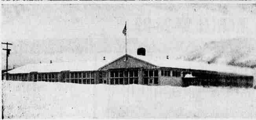
Headquarters — Top photo shows new Detroit Ranger Station on Highway 222 a mile west of Breitenbush bridge. Bottom photo shows new school now in use. Both buildings are built above the level of the reservoir to be formed by the reservoir back of Detroit dam. All buildings on the old Detroit townsite must be moved by June 1.
