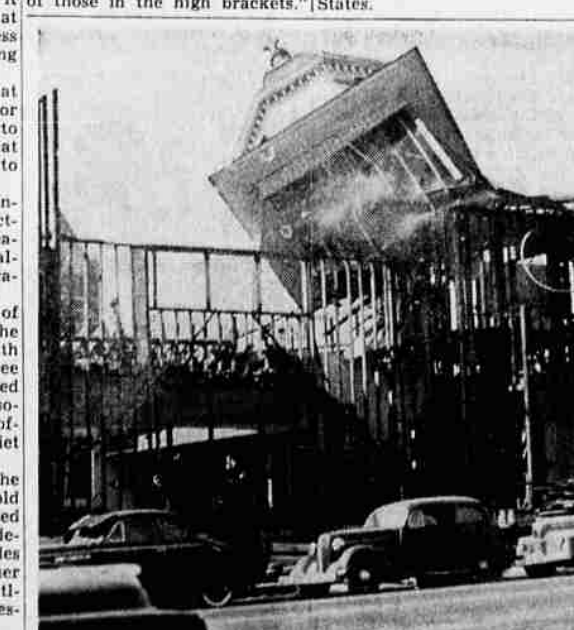
Falling Landmark—Steeple of old First Christian church at Church and High streets yields to wreckers as winch and cable pull it from the tower structure Thursday. The belfry once housed the chimes used to play sacred music daily. The room just below the steeple that collapsed also was known as the Belfry room and was used for children's Sunday school classes.
