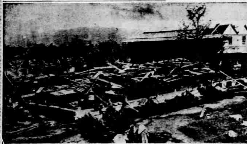
Where Hurricane Killed Eight—Splintered ruins is all that remains of one of the buildings at the Kingston, Jamaica, B.W.I. poorhouse where eight died in the worst hurricane in the British Island colony's history. Death toll for the island stood at 108. (APW/epphoto).
