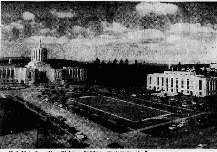
Mail Vista from New Highway Building—Photograph of capitol mall as made from the roof of the new highway office building affords this view of the capitol, sunken garden and the state library.
