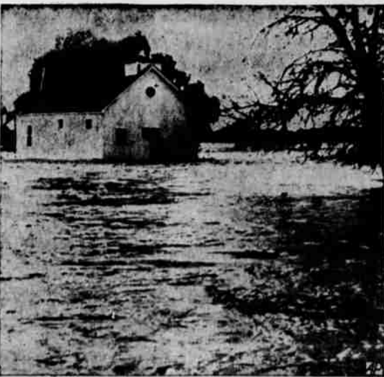
No Sunday Service—Services were suspended Sunday at this little Baptist church located near Centerville, Calif., when flood waters swept it from its foundation and deposited it a block away. Heavy rains and melting snow caused similar scenes in many sections of California. (AP Wirephoto)
