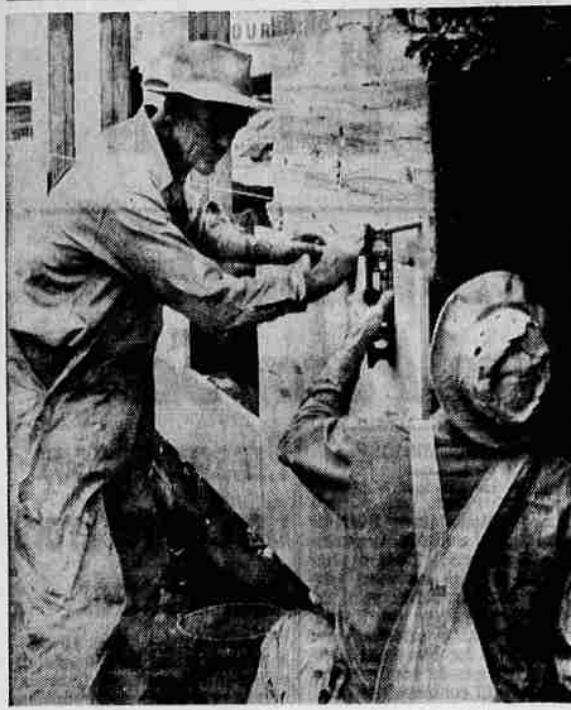
Marble Setters at Work on the new service station being constructed at the much disputed Capitol and Center street location. Sid Lofgren (left) and L. F. Skinner, employees of the Lutz Marble company of Portland are on the job. The station will open early in September.
