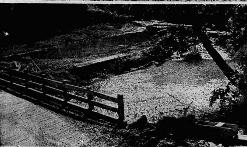
Channel Widened and Deepened to Control Luckiamute Flooding—Sharp bend in Little Luckiamute, where a new bridge on the Dallas-Kings Valley highway crosses the stream, receives a wider and deeper channel to prevent winter flooding. Approaches to the bridge have also been raised to prevent flood closing.
