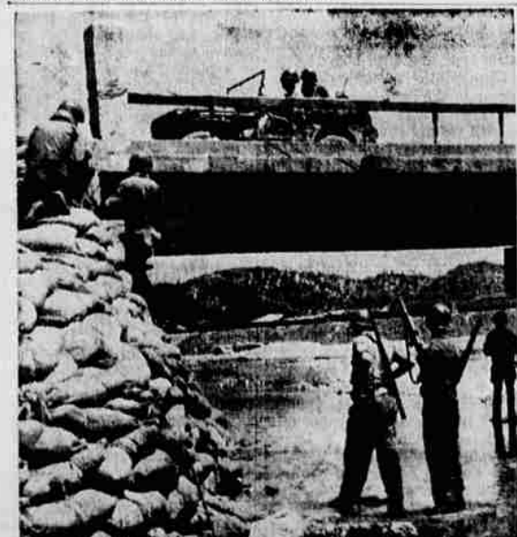
Bridge Busters—As a First Cavalry jeep rolls across a bridge near Yongdong, engineers connect wires to detonating charges to make sure the enemy doesn't get across. Other troopers stand by, on the lookout for snipers or a surprise attack. Photo by Ed Hoffman, NEA-Acme staff photographer. (Acme Telephoto)
