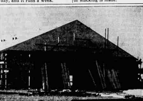
A Four Room Addition to the Washington grade school building is being rushed to completion for the opening of the 1950-51 term. The original building was completed only last October but because of the growth of the section around Lansing avenue and Silverton road an addition was found necessary. The contractor, T. J. Patzer, expects to have the addition completed on time. A two-room addition is also being made to the Swegle rural school.
