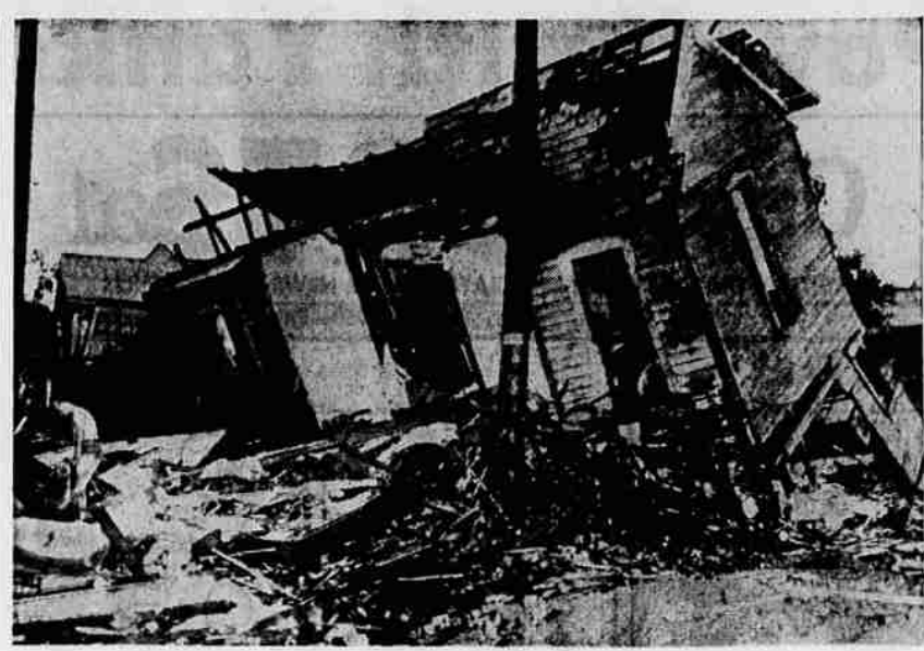
Tornado Damage—A resident of Lima, Ohio, sifts through the wreckage of his home (left) after a tornado tore through an area 20 blocks long and four blocks wide in the city of 50,000 population. One person disappeared during the touch-and-go tornado, 38 were injured and damage was estimated at $50,000. (Acme Telephoto)
