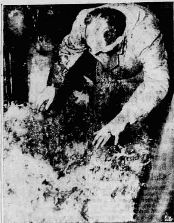
Neither Snow Nor . . . —A New York newspaperman struggles through a cascade of water pouring down stairway on 12th floor of New York's Woolworth building in lower Manhattan on his way to cover fire which burned out part of the 23rd floor of the building—once the city's highest structure and a mecca for tourists for nearly 40 years. It is a 60-story building. (AP Wirephoto)
