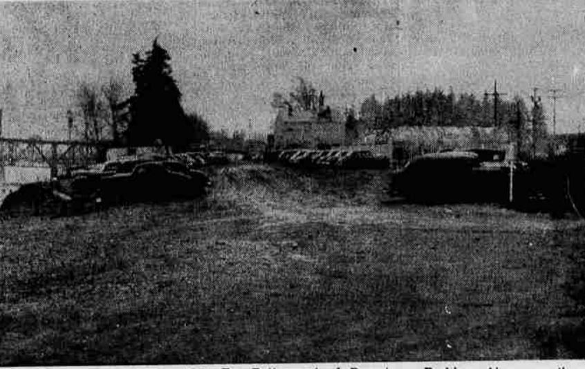
For Betterment of Downtown Parking —Above, another section of Liberty street, between State and Ferry, which Mayor Elfstrom recommends be widened to provide angle car parking and increase facilities. Below, River street between Court and Center, recommended for improvement as free parking area.
