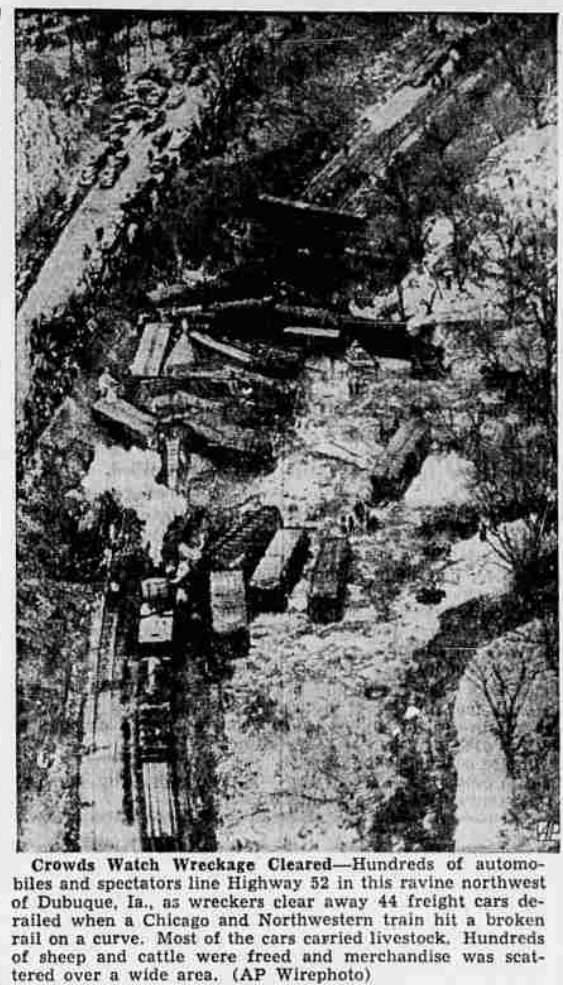
Crowds Watch Wreckage Cleared—Hundreds of automobiles and spectators line Highway 52 in this ravine northwest of Dubuque, Ia., as wreckers clear away 44 freight cars derailed when a Chicago and Northwestern train hit a broken rail on a curve. Most of the cars carried livestock. Hundreds of sheep and cattle were freed and merchandise was scattered over a wide area. (AP Wirephoto)
