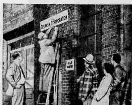
5. "HELP WANTED" sign went up fast. "The Delman Corporation" rented factory space, hired 12 employees (mostly ex-G.I.'s), learned what Ford teamwork means. Ford Engineers helped them plan manufacturing operations. Ford Purchasing helped get machinery, materials. Soon The Delman Corporation was a going concern.
