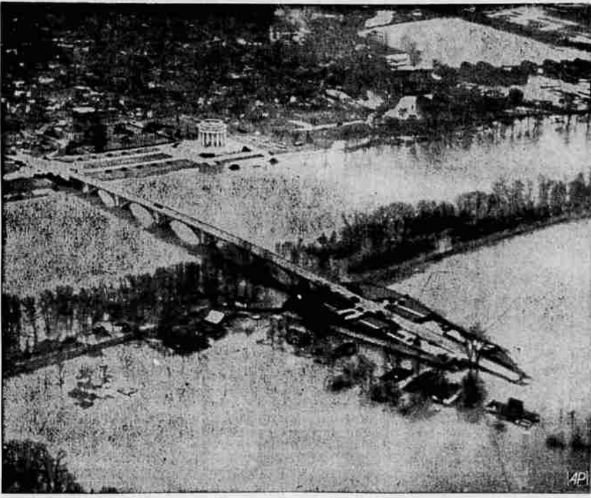
Wabash Flood Covers Highway—U. S. highway 50 dips far under the Wabash river floodwaters near the west end of the bridge opposite flood-besieged Vincennes, Ind. The breached Russell-Allison levee is shown dividing the waters. The classic columns of the George Rogers Clark Memorial are shown on the Vincennes waterfront (center, foreground). (AP Wirephoto)
