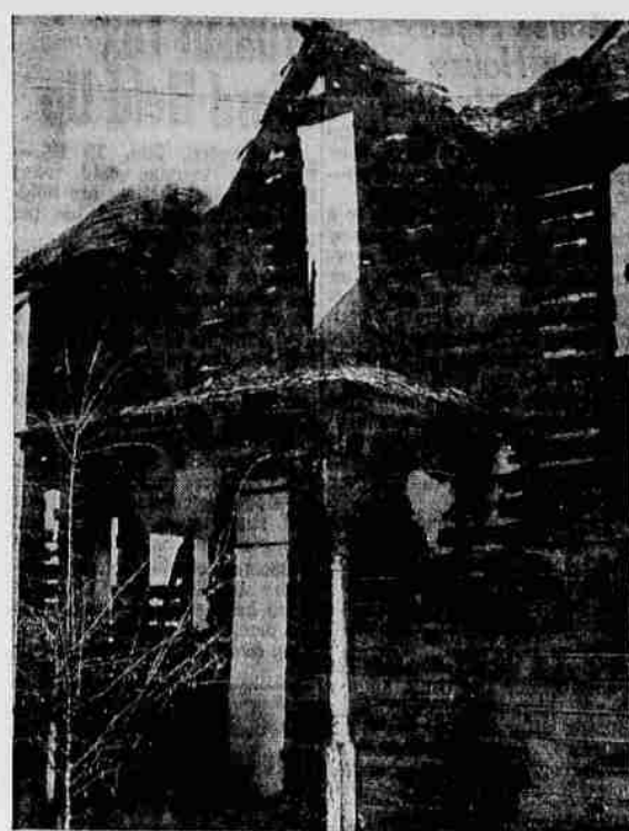
Fire Hits Silverton—The Charles Case home in Silverton at 701 N. First street was completely destroyed by fire recently with the family forced to flee in their night clothing. Case, who was seriously burned in leading his wife and children to safety, is in the Silverton hospital. Friends are providing clothing for the family. (Photo Silverton McEwan shop).
