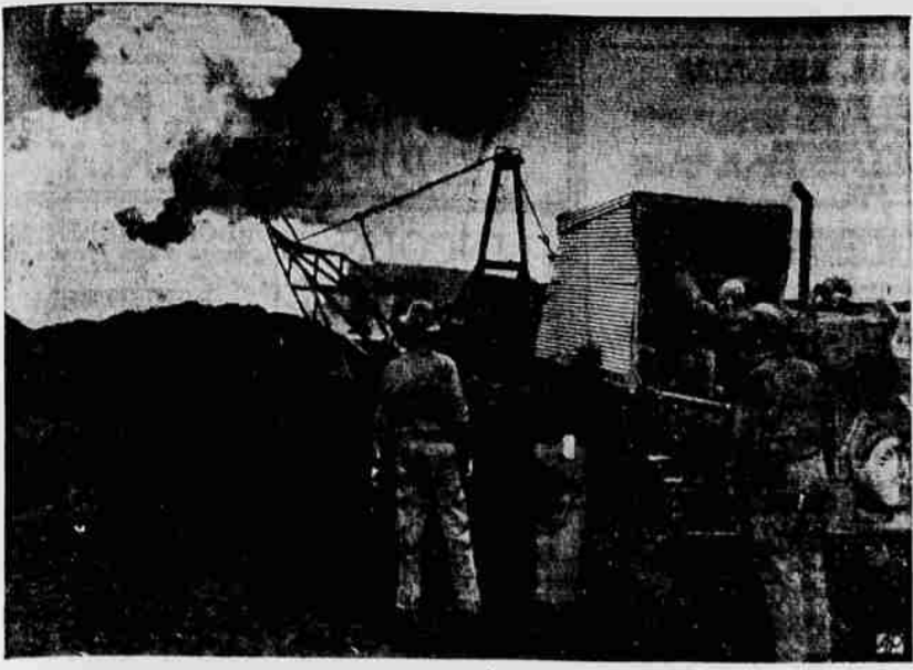
Let 'Er Blow!—That's 200 pounds of nitroglycerin on the end of that weird-looking apparatus. The explosive was detonated over the mouth of a blazing oil well at Elk City, Okla., and snuffed out the flames for 10 minutes. However 100-foot flames sprang up again from the well, ignited by a gas explosion. Further attempts to extinguish the fire will be continued. (AP Wirephoto.)
