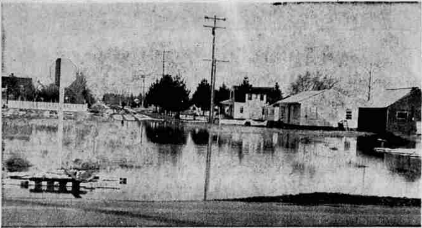
Loblolly at Four Corners —The above picture shows the unhealthful and inconvenient condition on Mahrt avenue at Four Corners, caused by wet weather. Residents say they can get no official action for their relief, and at the same time are not permitted to do the work themselves.
