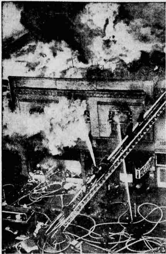
$200,000 Fire—Smoke and fire is shown billowing from the Kramer Carlton & Printing company and the Green hotel at the height of a blaze which destroyed the structures at 421 J street, Sacramento, Calif. At least eight persons, including five firemen, were injured. (AP Wirephoto)
