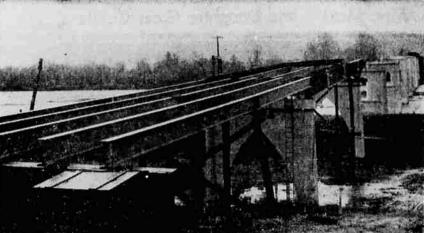
Delayed Bridge Gets First Steel - Independence bridge spanning the Willamette, scheduled for completion before January 1, has received steel girders and stringers on piers 9 and 10. No workmen are now employed on the job and no additional steel will be laid until the spring of 1950
