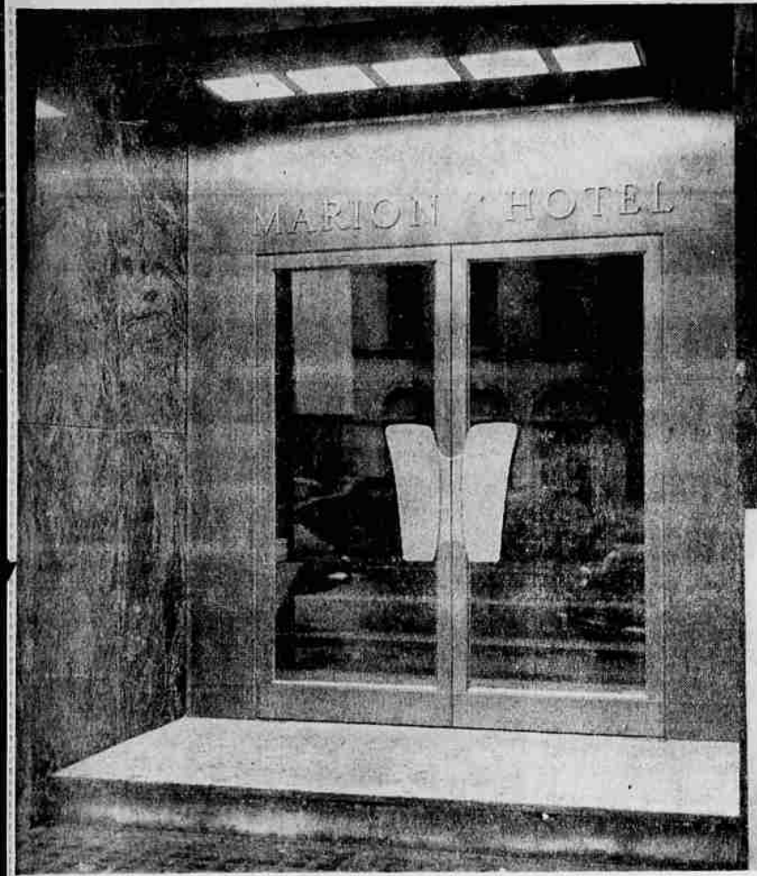
Outstanding Entrance Features Remodeled Marion—Commercial street entrance for Marion hotel now being remodeled features Virginia marble and doors costing approximately $2000 each. When completed sometime next week this outstanding entrance will represent an investment of near $7000.
