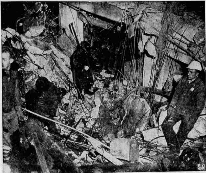
Probs Wreckage for Dead —Firemen and rescue workers use hack saws to cut away the debris as they probe the ruins of Swift & Company's main office building at Sioux City, Ia., seeking additional victims of an explosion which rocked the plant. At least 16 persons were known dead and scores of others were injured. (AP Wirephoto)
