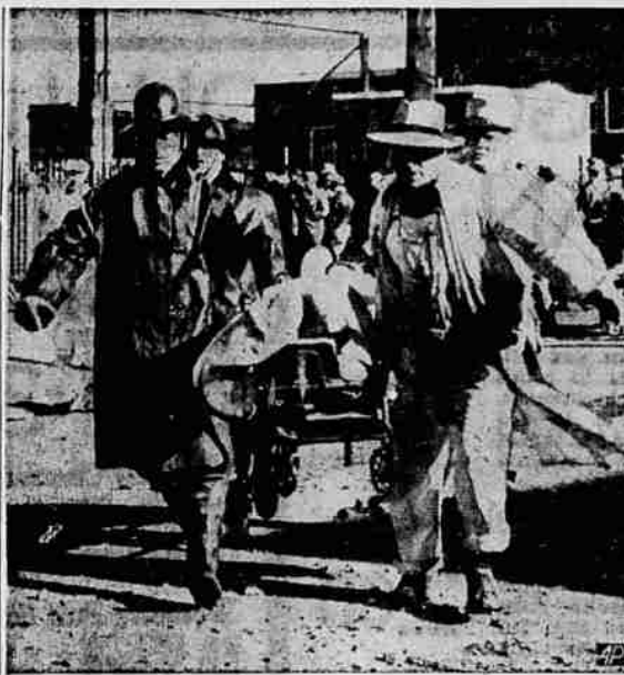
Body Removed from Wreckage—Firemen carry a body from the blasted office building of the Swift & Co. plant at Sioux City, Ia., after an explosion turned parts of the building to a shambles. (AP Wirephoto)
