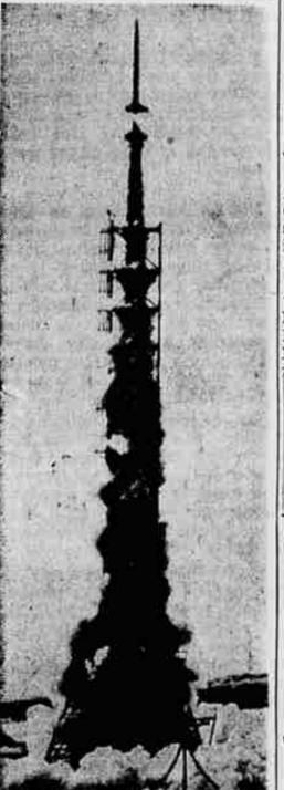
**High Flyer**—Air Force Aerobee, upper-atmosphere research rocket, soars skyward from launching tower at Holloman air force base, Alamogordo, N. M., attaining an altitude of 60 miles above the earth. One of 60 such rockets to be launched in a two-year program of atmospheric research, this particular rocket is 20 feet long, about one foot in diameter and has three fins to provide stability. (Acme Telephoto)
