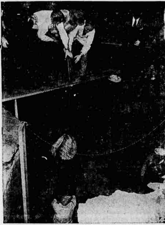
Cave-in Victim —Rescue workers pull the body of John Cipriani, 30, Monterey, Calif., laborer, to the surface from cave-in where he was killed while working on a sewer construction job at Carmel, Calif. A second man, Carl D. Simon, 25, of Monterey, was also in the cave-in but rescue workers reached him in time to save his life. (AP Wirephoto)
