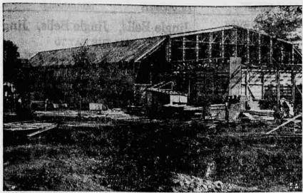
Portable Theater-The Alu-Palast (above) in Hamburg Germany, is an aluminum portable theater with a stage 40 by 66 feet and seats for 1,200 and can be assembled in 12 c
