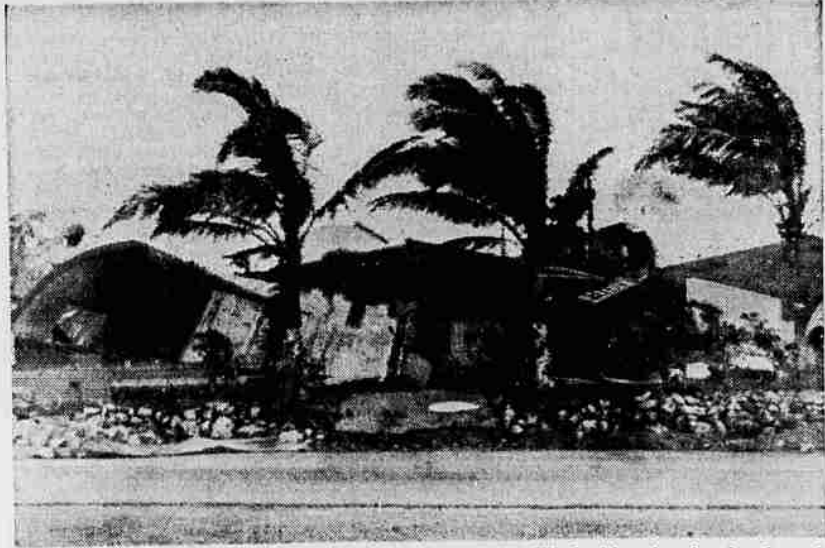
Typhoon Lashes Guam—Wind-whipped palm fronds and demolished quonset huts (background) graphically show the force of the 145-m.p.h. typhoon which hit Guam, causing damage expected to run into millions of dollars. No deaths were reported as a result of the typhoon. (Navy Radiophoto via Acme Telephoto)
