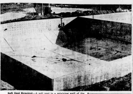
Soft Spot Repaired-A soft spot in a retaining wall of the 3,000,000 gallon water reservoir at Dallas was revealed when first checks were made. Repair of these and a few leaks to be stopped will delay completion of the huge tank another ten days, according to E. L. McCleary, water commissioner. (Photo by Abel.)
