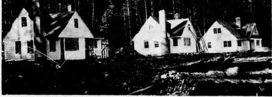
Housing facilities for hatchery attendants now almost complete.
