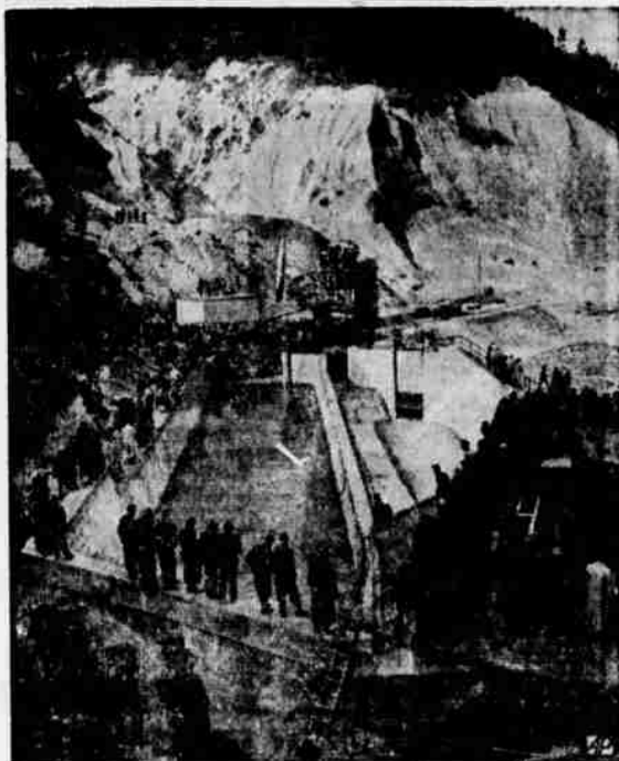
Power for Germany —Waters of Riss creek are dammed to flow through a 4½-mile tunnel under two mountain ranges to Walchen Lake near German Tyrol border. It will increase Lake's power production by 100,000,000 kilowatts a year.
