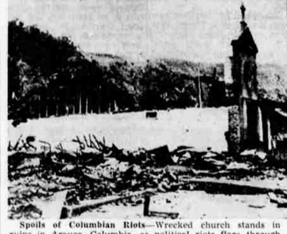
Spoils of Columbian Riots—Wrecked church stands in ruins in Arauca, Columbia, as political riots flare through the country, leaving a wake of ruined buildings and heavy casualties. The newspaper El Liberal reported that rioting at one point had reached the proportions of a "pitched battle." The pre-election riots have claimed some 300 lives. (Acme Telephone)
