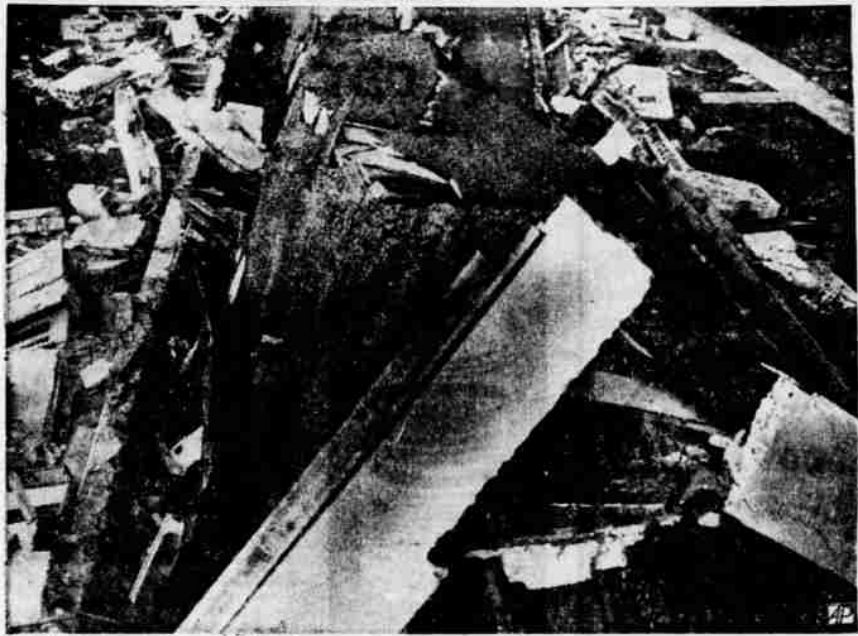
Explosion Injures 14 —What was once a two-story, four-family apartment unit at a federal housing project in Dallas, Tex., lies almost level with the ground after an explosion blasted the building into rubble, injuring 14 residents. An accumulation of leaking gas was blamed for the explosion. Authorities said it was a miracle that none of the occupants were killed in the blast. Below—Another view of the aftermath of the explosion. The walls went outward and the roof collapsed.
