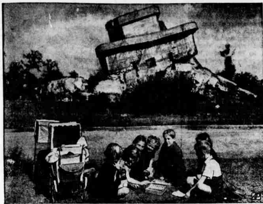
Play Near Bomb Shelter—Youngsters play in the shadow of one of the largest Berlin bomb shelters. The walls, 12 feet thick, were wrecked by three charges of explosive.
