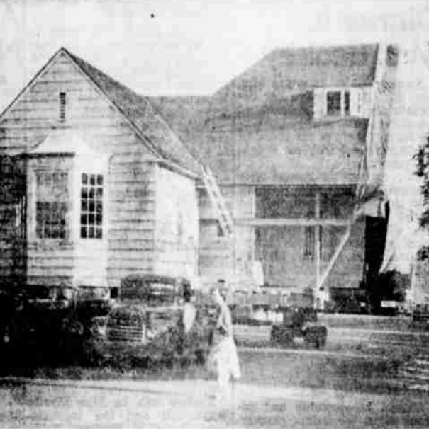
Eyre House Moved to New Location —David Eyre's home, formerly located on Summer street where the state will soon construct a new office building for the highway department, has been bisected and one section is shown in the process of being removed to a new location at Mission and High streets. H. Henkel & Son, Portland movers, report the section rapidly transported to the new site on three dollies weighs about 30 tons. The remaining section will be moved in a few days. Harry Dorman purchased the house and it is the only one of many on the block to be moved.
