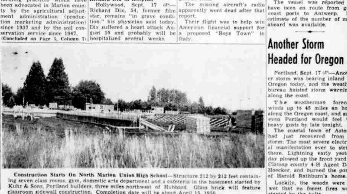
Construction Starts On North Marion Union High School—Structure 212 by 212 feet containing seven class rooms, gym, domestic arts department and a cafeteria in the basement started by Kuhr & Sons, Portland builders, three miles northwest of Hubbard. Glass brick will feature classroom sidewalk construction. Completion date will be about April 15, 1950.
