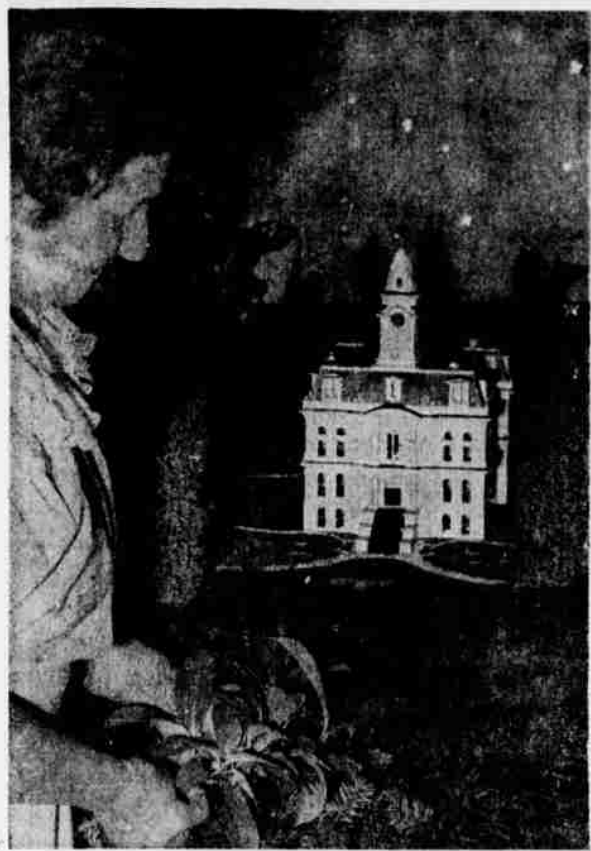
Miss Renska Swart and the model of the Marion county courthouse she displayed at the Oregon State Fair last week gathered over 1000 signers to her petitions seeking to keep the old structure intact at its present location. She would have most of the county business transacted in a business building on another site leaving the courts on the main floor of the present structure and the upper floors used for county museum purposes. The courthouse model was made some years ago at the behest of the late C. P. Bishop who furnished the funds.
