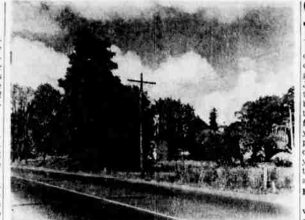
Site for Proposed West Salem Shopping Center —Frontage of a 16-acre tract facing Edgewater street between Senate street and Cascade drive tentatively allocated for a shopping center 350 feet wide and about 300 feet deep. Behind this area, in one two, would be courts and a recreational center. Eight acres, classified as zone one, would be devoted to residential view property and scenic drives. Ground plans are being prepared by Lyle Bartholomew, architect, and Walter Musgrave, mayor of West Salem, is handling the development for Francis Smith, property owner.
