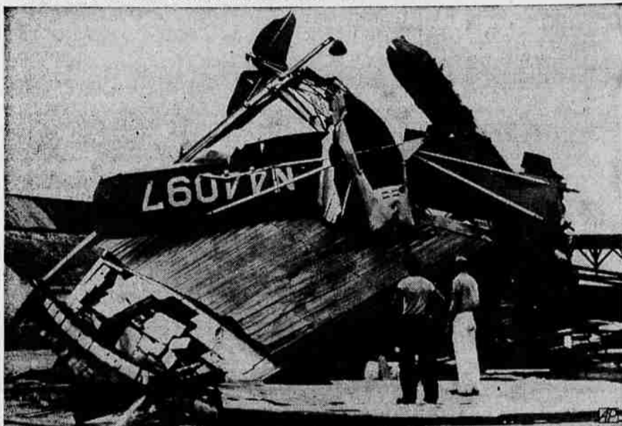
Hurricane Wrecks Planes—One of the 37 airplanes wrecked by the hurricane hangs atop wreckage of its hanger at West Palm Beach, Fla. Homes were twisted into matchwood by winds that reach a velocity of 160 miles an hour. Highways clogged with rows of snapped and twisted trees. Damage will run into the millions of dollars. It will exceed by far the historic disaster of 1928 that took upwards of 2,000 lives. (AP Wirephoto)
