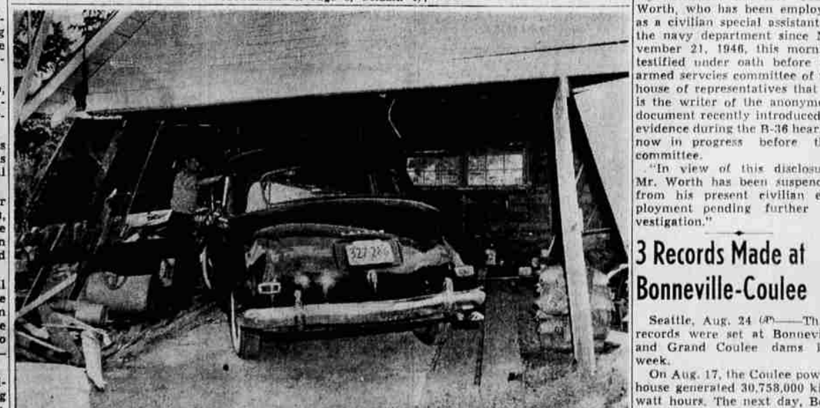
Car and Garage Damaged—Pictured here is damage caused to car and garage of W. S. Brown, 1840 North Summer street, caused by car getting out of control as Mr. Brown drove into the Garage Monday night. His foot slipped off the brake pedal and hit the foot throttle, causing the car to lunge out of control. Before hitting the garage wall the car collided with a lawn swing and the house. The man in the picture is not Brown, but a man from a service garage.
