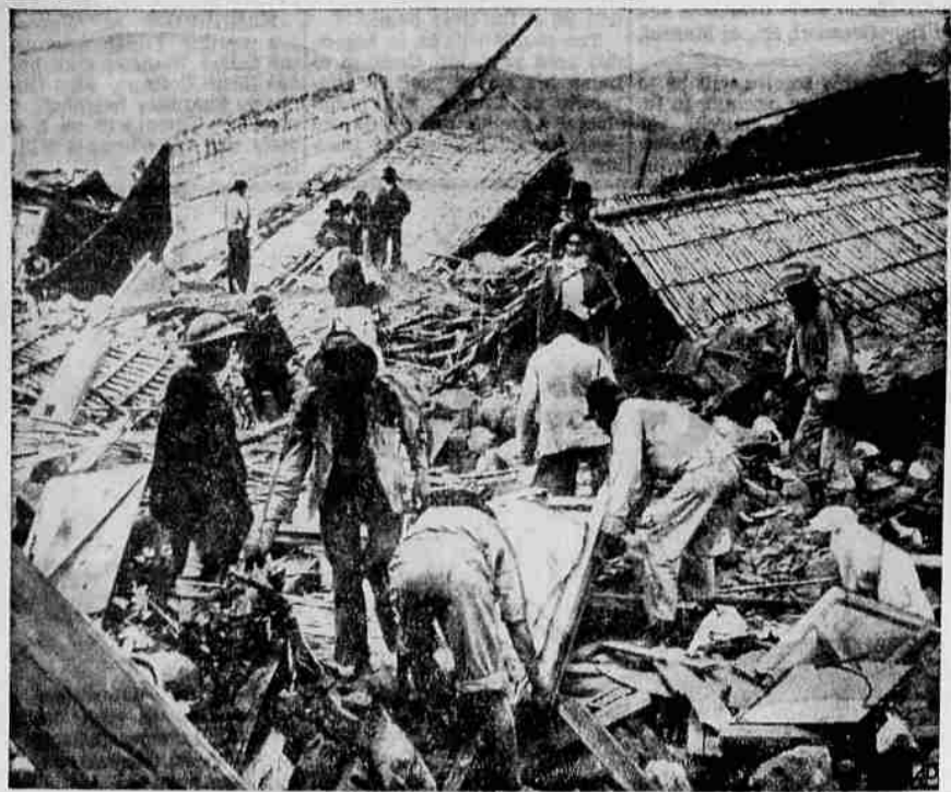
Digging Out the Dead —Survivors of the Ecuadorean earthquake dig out their dead from the ruins of the town of Pelileo. Hundreds died amid such desolation. Violent earth movement shook off plastered walls and tiled roofs and collapsed the homes. (AP Wirephoto)
