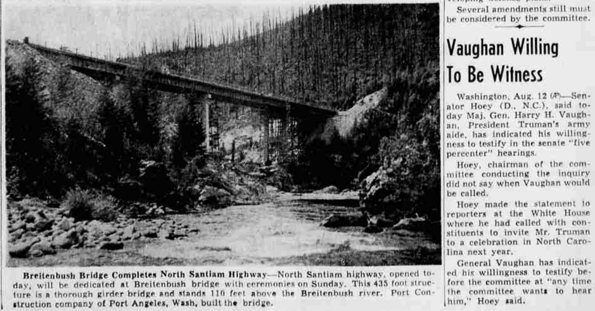
Breitenbush Bridge Completes North Santiam Highway —North Santiam highway, opened today, will be dedicated at Breitenbush bridge with ceremonies on Sunday. This 435 foot structure is a thorough girder bridge and stands 110 feet above the Breitenbush river. Port Construction company of Port Angeles, Wash., built the bridge.
