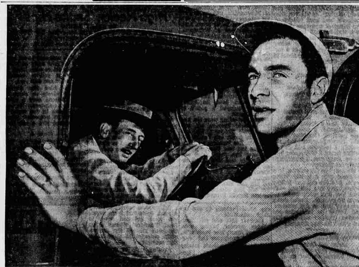
These telephone men will soon make a damaged long distance cable carry calls again. Come along and see how it's done.
