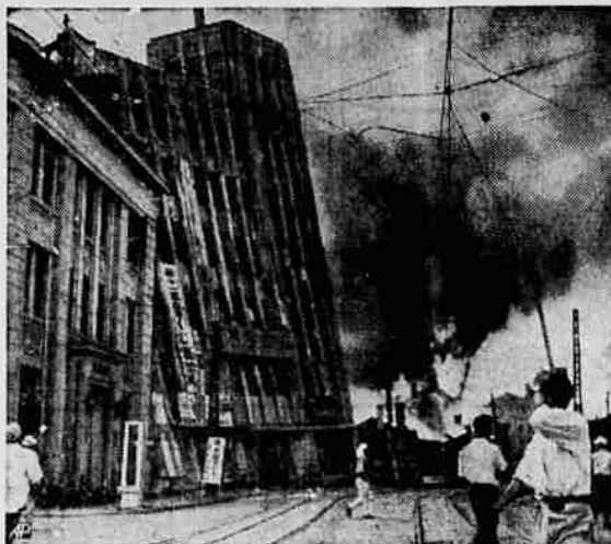
Leaning Over Backward this Fukui building was wrecked.
