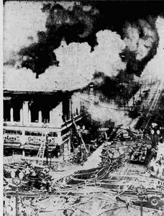
Gambling Club Damaged by Fire —A three-alarm fire gutted the second story Sportsman's club in Portland, Ore., causing heavy damage to eight shops in the two-story brick building. Damage was estimated at $100,000. (Acme Telephone photo.)
