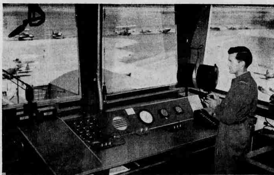
Tower Controls Airport Ground and Air Traffic—Charles Huggins, one of six operators who man the control tower 24 hours a day, at Salem airport, directs air and ground traffic through an eight-hour shift. Control devices shown in the tower are, from left: the speaker control panel, spotlight control handle, large speaker, altimeter setting indicator, wind direction and speed indicator and the light control panel.
