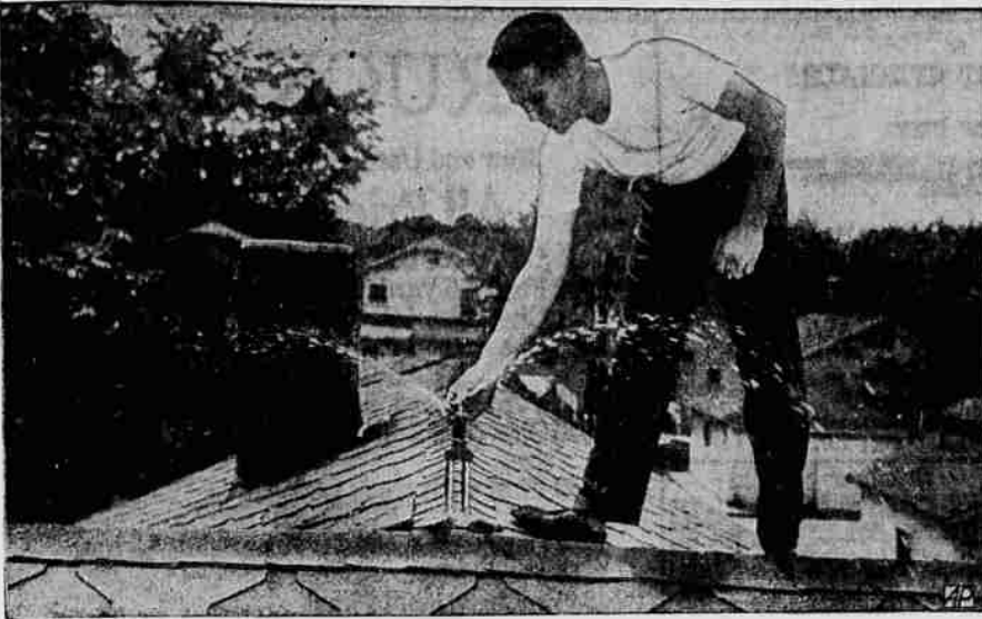
Beating the Heat —Robert A. Todd (above) is shown adjusting a revolving lawn sprinkler head atop the roof of his Dayton, Ohio, home to cool the inside. An ordinary length of garden hose and sprinkler is used. In preliminary tests the temperature dropped from 92 to 84 degrees. "If you began the spray when the roof is still cool, you've got a head start in whipping rising temperatures," Todd claims. (AP Wire-photo)
