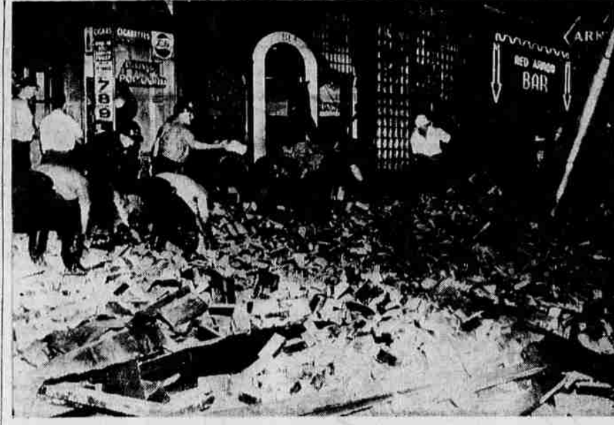
Building Front Collapse Kills Four—Firemen and rescue workers clear the rubble of bricks that crashed to the street in Pittsburgh, Pa., killing four persons and injuring eight, four critically. A large neon sign weakened and collapsed the brick parapet atop the one-story building, showering the bricks onto the street below. (Acme Telephoto)
