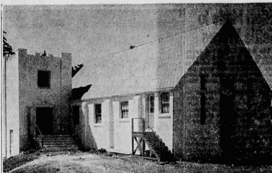
New Liberty Christian Church to be Dedicated Sunday—First services in this new Liberty church will be the dedicatory ceremony Sunday afternoon at 3 o'clock. Rev. E. A. Parrish, pastor. The structure of pumice block construction is 28 by 60 feet and contains five rooms besides the large auditorium and a full basement.
